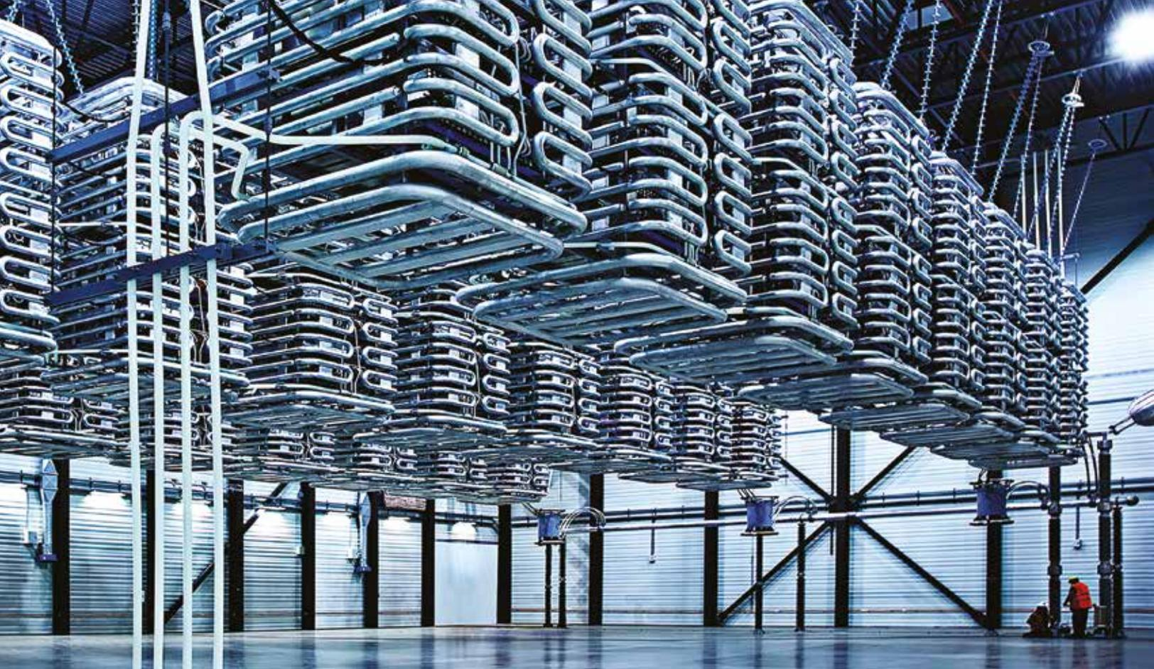
asynchronous HVDC connections are often the only practical way to join systems operating at different frequencies or where it is not possible to make a direct link.
